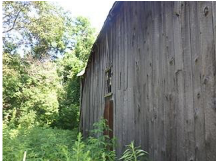
Photo 2-4 Sidewall kick out and in, near failure.
