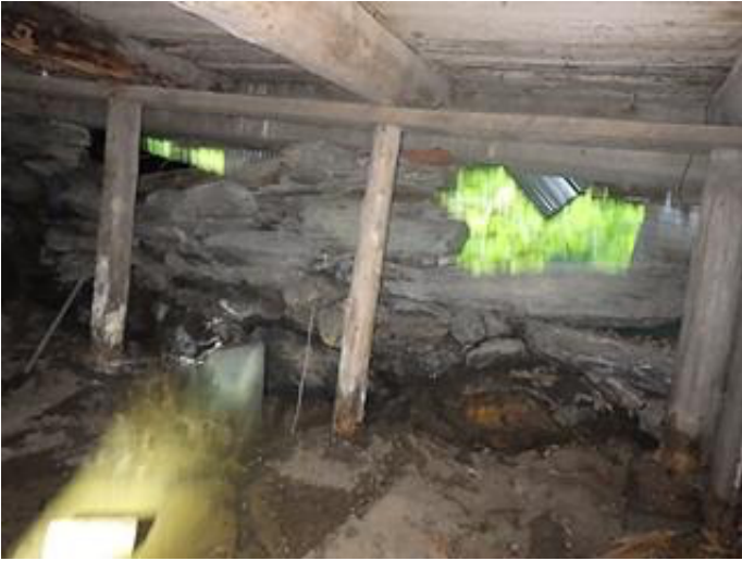
Photo 2-16 Voids in the stone foundation, rotten supports.
