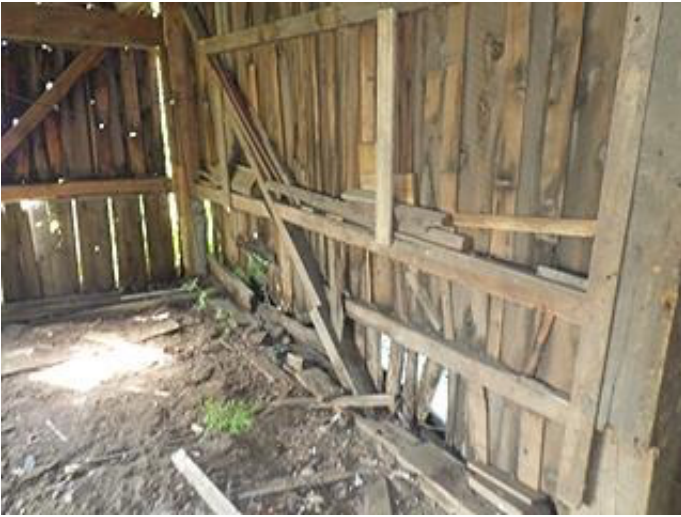
Photo 2-21 Siding damage and or missing throughout the barn.
