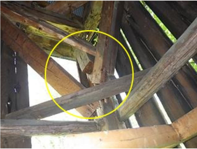
Photo 2-6 The NE corner post is rotten/decayed and pulled apart. In failure, possible for collapse.
