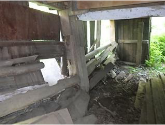
Photo 2-5 Vertical support is ready to kick out below the prior photos.
