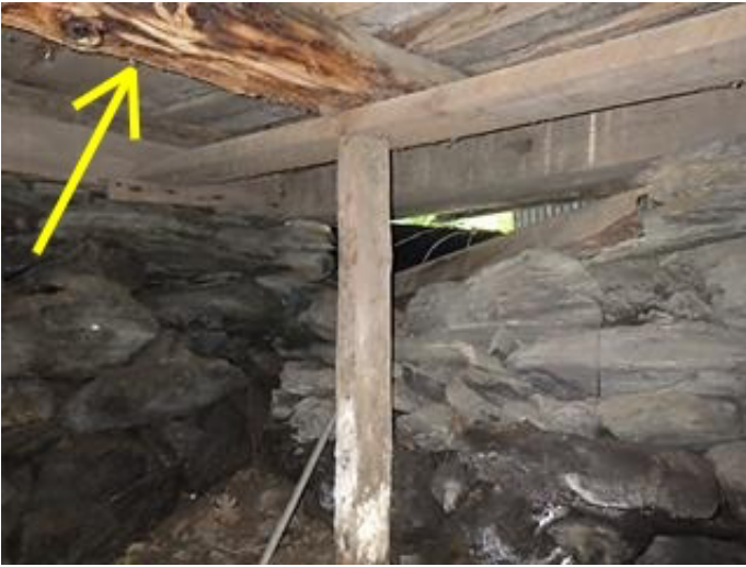
Photo 2-13 Multiple areas of rot and decay.
