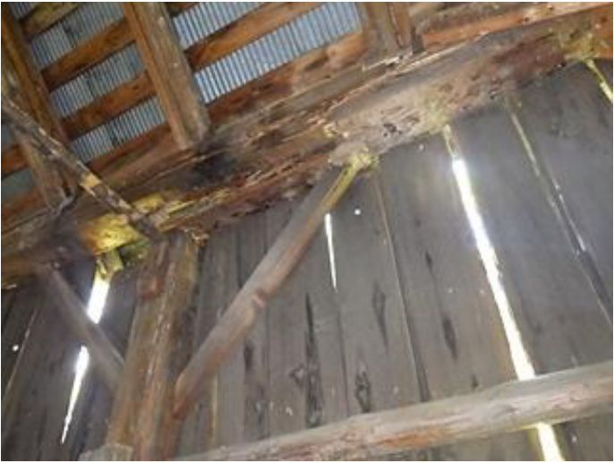
Photo 2-18 Rotten decayed areas near the middle support post, north side.
