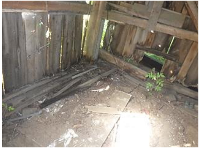
Photo 2-22 NW corner base plate disintegration.
