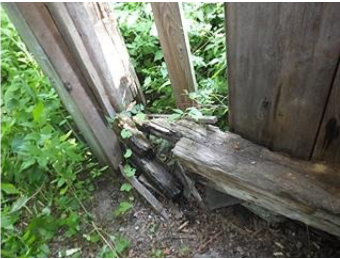
Photo 2-9 Base plates are decayed and or disintegrated into the soil. NE corner
