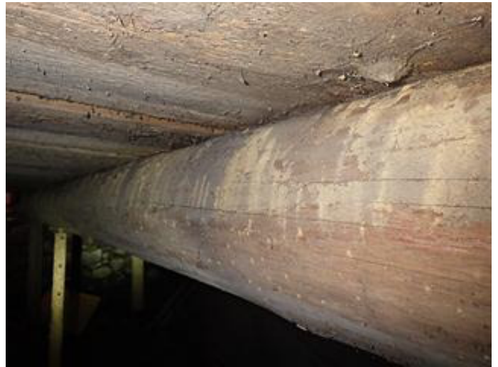
Photo 2-24 Active powder post beetle activity throughout the barn, wood-destroying insects.
