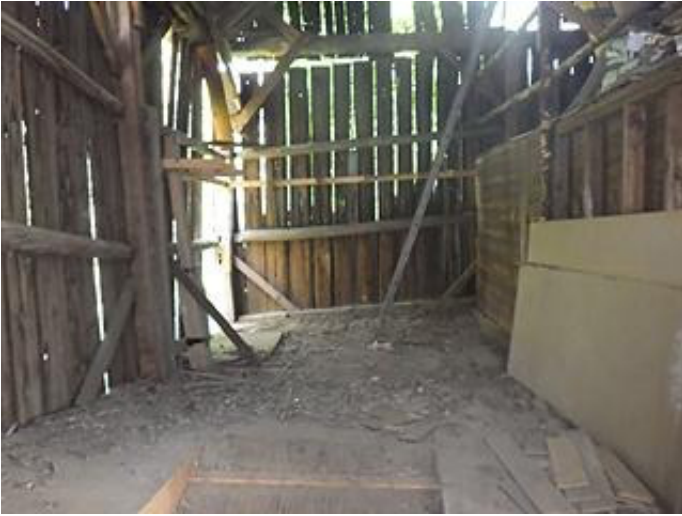
Photo 2-8 The floor is twisted and unstable.
