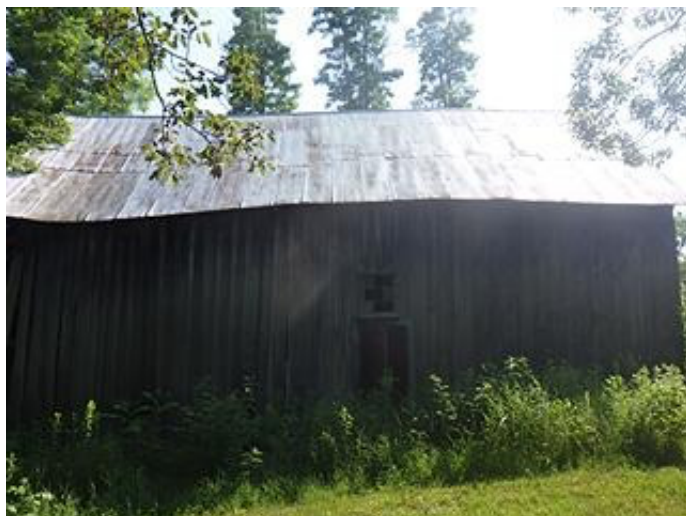
Photo 3-3 Structural support failures translate to the roof system, very dramatic deflection was noted.
