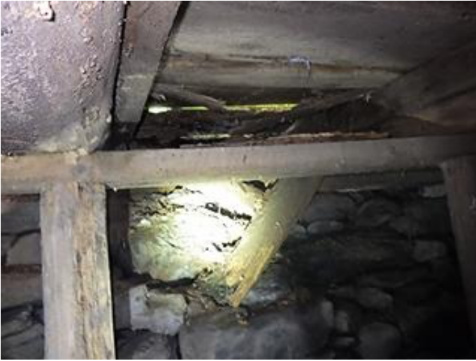
Photo 2-15 Floor decking decay, has fallen through.
