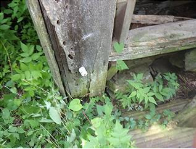
Photo 2-19 Rotten corner post.
