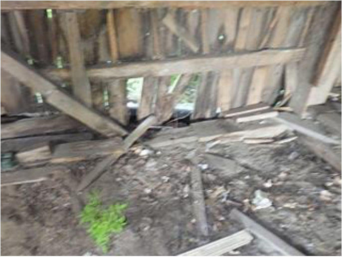
Photo 2-20 West side base plate decay.
