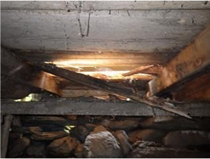
Photo 2-14 Floor rot and decay in multiple areas.
