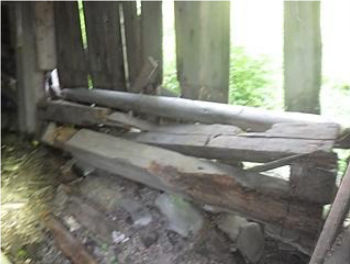
Photo 2-11 The base plate has no structural integrity.
