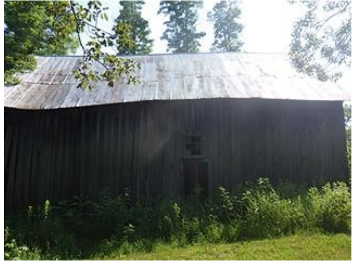
Photo 2-2 Structural support failures translate to the roof system, very dramatic deflection was noted.
