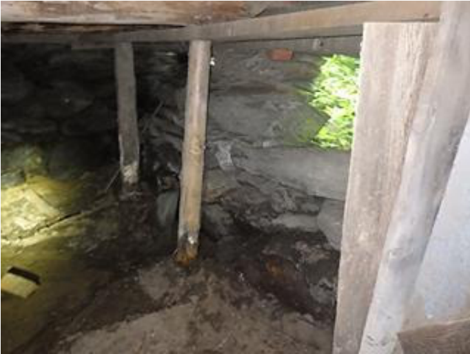
Photo 2-12 Most vertical supports are out of plumb, decayed at their base.
