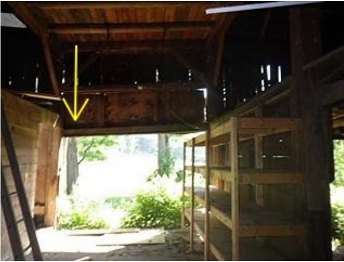
Photo 2-17 Wagon bay opening deflection due to structural failures.
